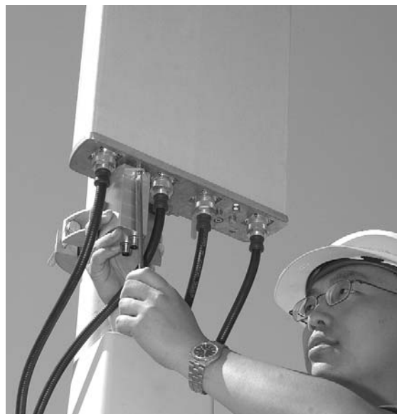
Antenna Control Unit being fitted to an antenna
